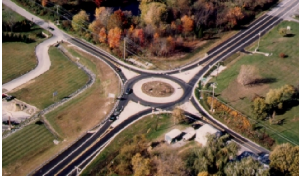
Figure 1 Views of Roundabout in Cecil County, MD
